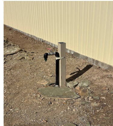
Photograph 7 - Standpipe from the rain water tank at the side of the shed.
