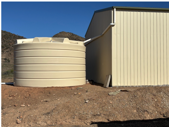
Photograph 6 - Rain water tank in place next to the shed.
